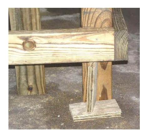
Once I had the frame in place I fastened it to the potting bench legs using 2-1/2" screws. I drilled pilot holes first to make inserting the screws easier. Once again, make sure the legs are plumb before fastening permanently.
