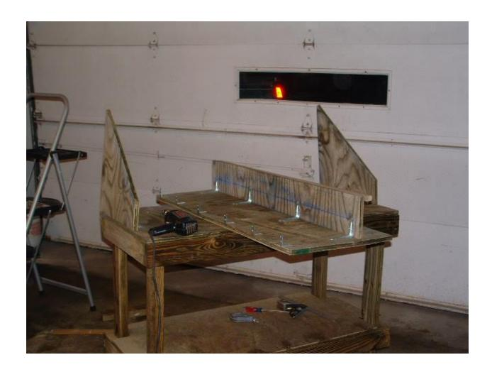
Now slide the back of the potting bench between the two side pieces you just installed, allow it to rest on the top of the potting bench. Secure in place with 1-5/8" screws. After securing the back of the potting bench to the top and sides, put one screw through each side into the top shelf, giving the shelf additional support.
