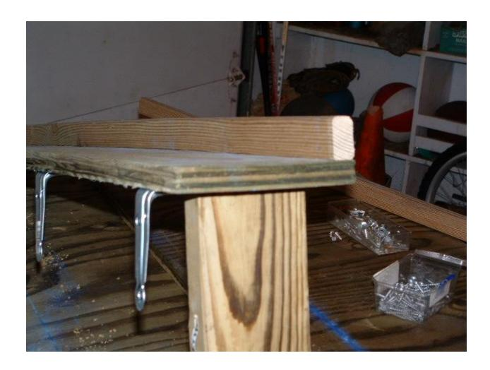
On the opposite side of the top shelf install the four 4" by 5" shelf brackets as shown in the above photo. Just space the four brackets along the length of the shelf.
