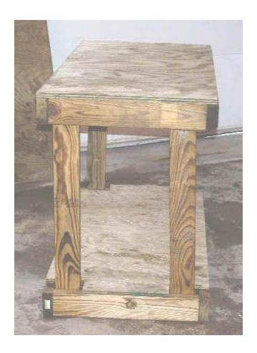
Carefully set the top of the potting bench over the legs as shown above.
